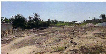
Church construction at Shama
