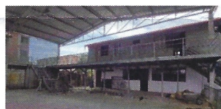
Mezzanine Under Construction
