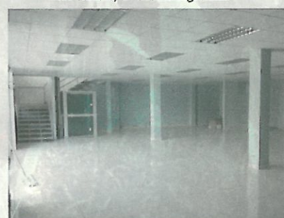
Fig. 6 – Photo Looking at stair and elevator at first floor
